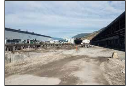
Potroom 1 structure removed
