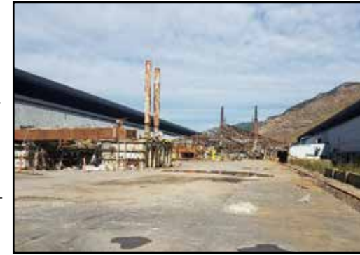
Former casthouse removed
